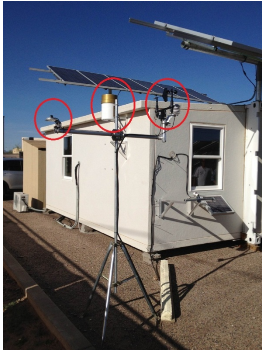
Figure 2.2.2: 2 meter tower installation for Solar Radiation, Wind Speed and Direction, Precipitation, and Outdoor Air Temperature, approximately five meters southwest of the structure. Prevailing winds are from the west during the day and the east at night.
